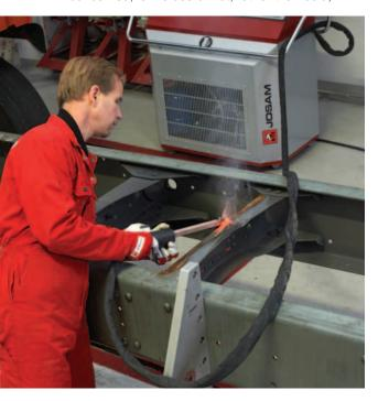
straightening, advises Paul 'Toby' Talbot, accident repair centre manager at Keltruck's West Bromwich site. The Scania dealership, which also operates a repair centre at a site in Newark, has started using an induction heating system, sourced from Josam, to help bring chassis back into line.
